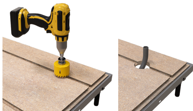
Drilled hole in HeatFloor 22. LK Conduit pulled up through the hole.
